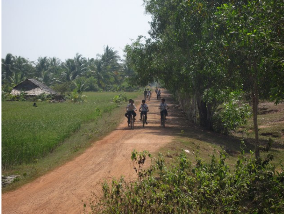
Internal commune road linking villages within the commune to the local school and other roads that lead to another district.
