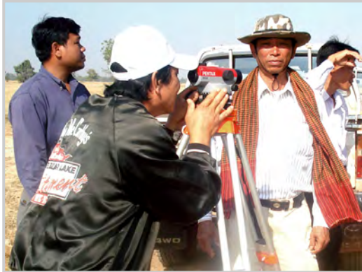
Surveying activity before construction
