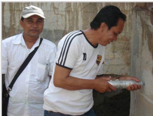
Culvert concrete testing activity
