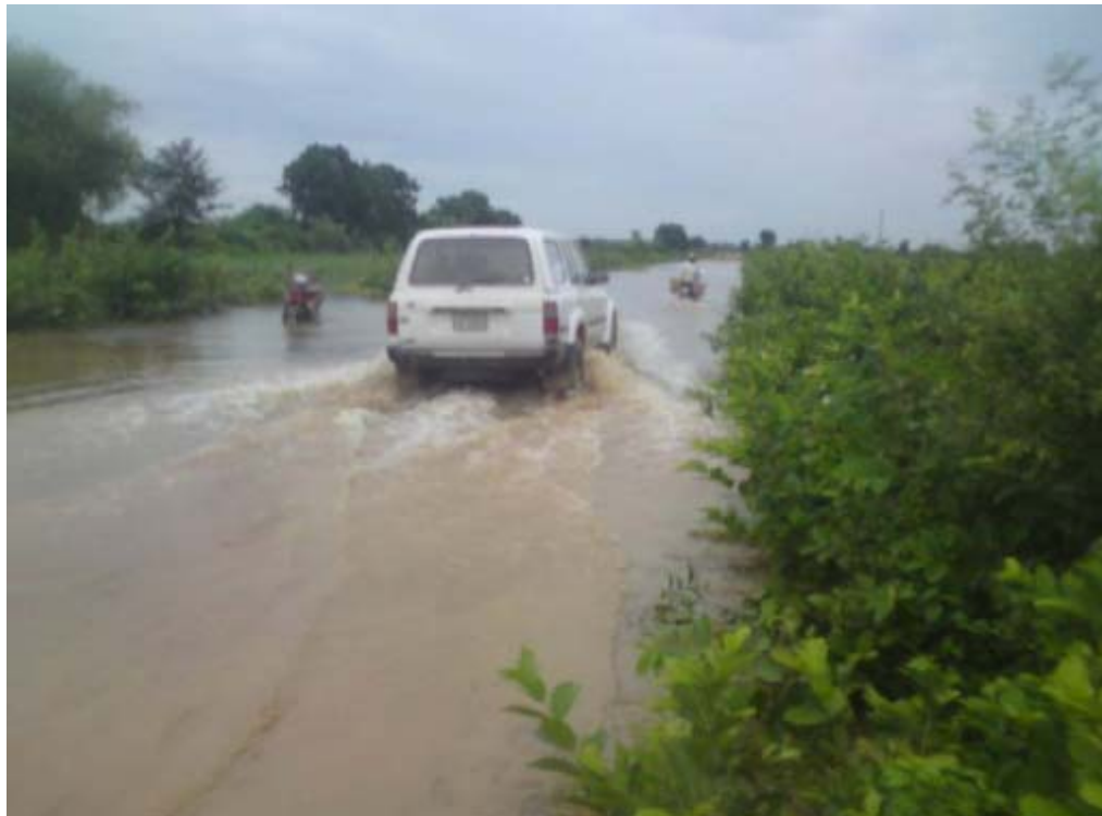
Road to communes were flooded with rain water
